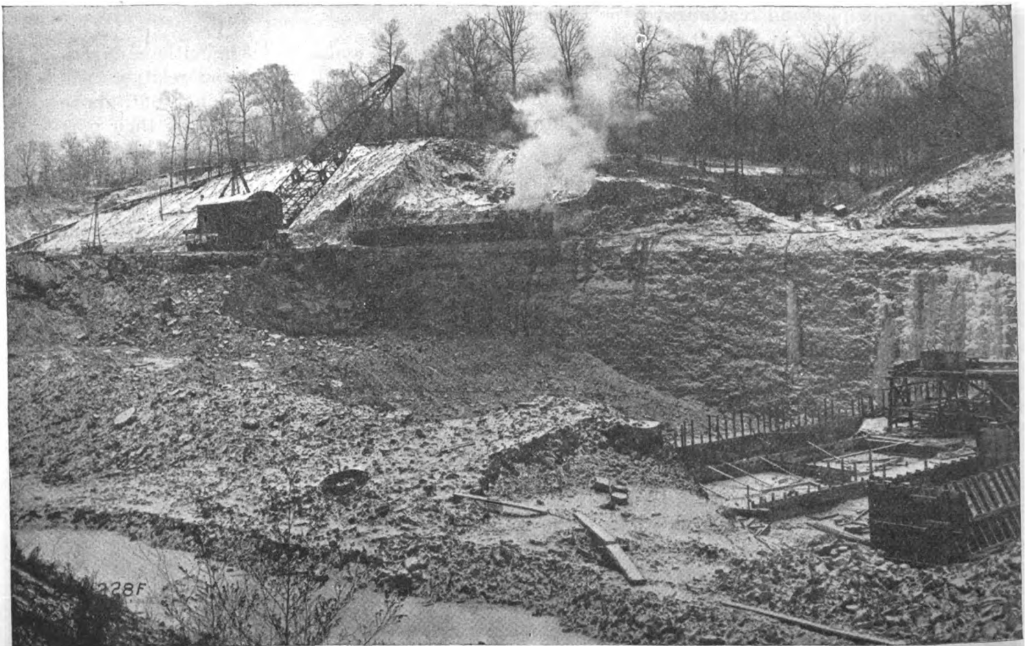
Excavating for outlet structure at Taylorsville Dam. Dragline machine excavating a rock sixty feet in depth. Following up excavation with concrete work (extreme right)
