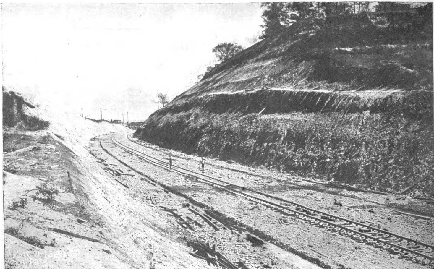
Railroad cut at Huffman Dam to carry the Big Four and Erie railroads around the dam and retarding basin. This is a view of the excavation looking toward the east
